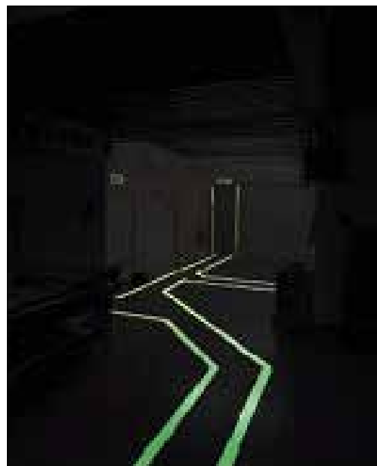
Figure 53: A 'way-guidance' system
